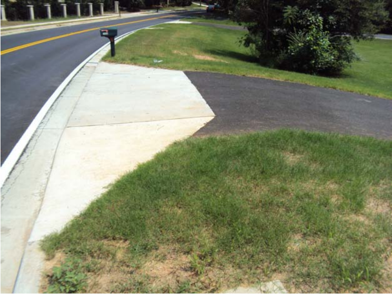
Figure 10: Concrete Driveway Apron
