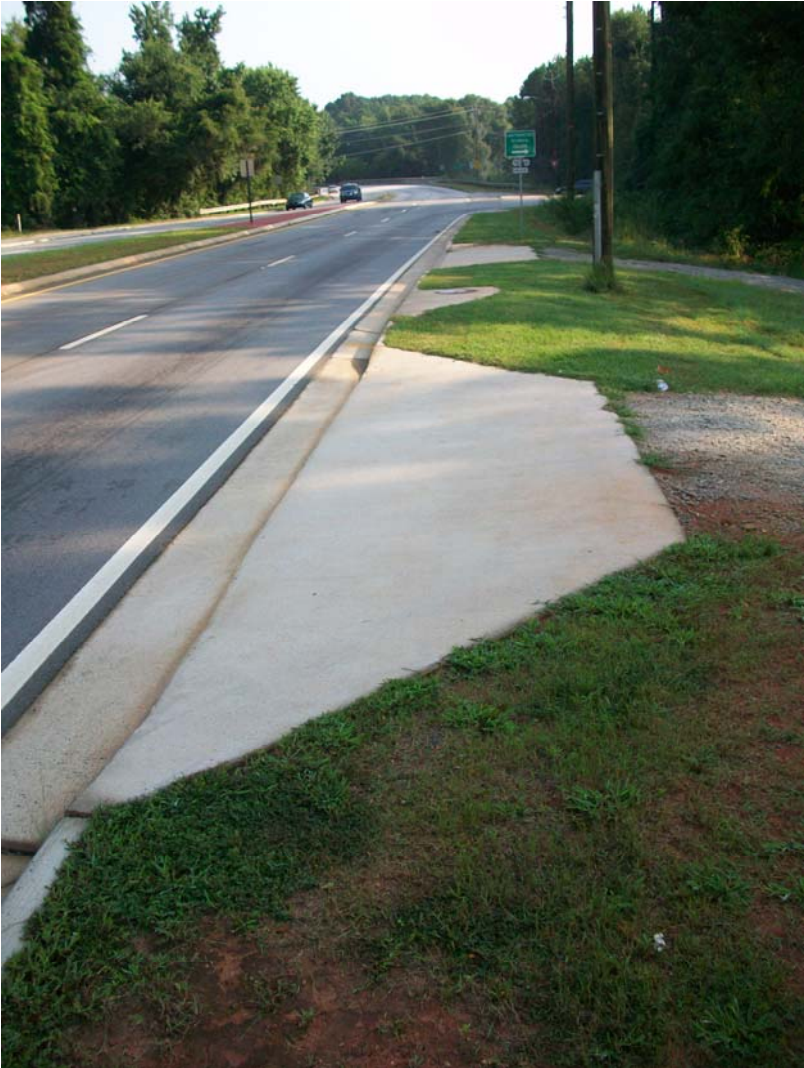
Figure 8: Concrete Driveway Apron
