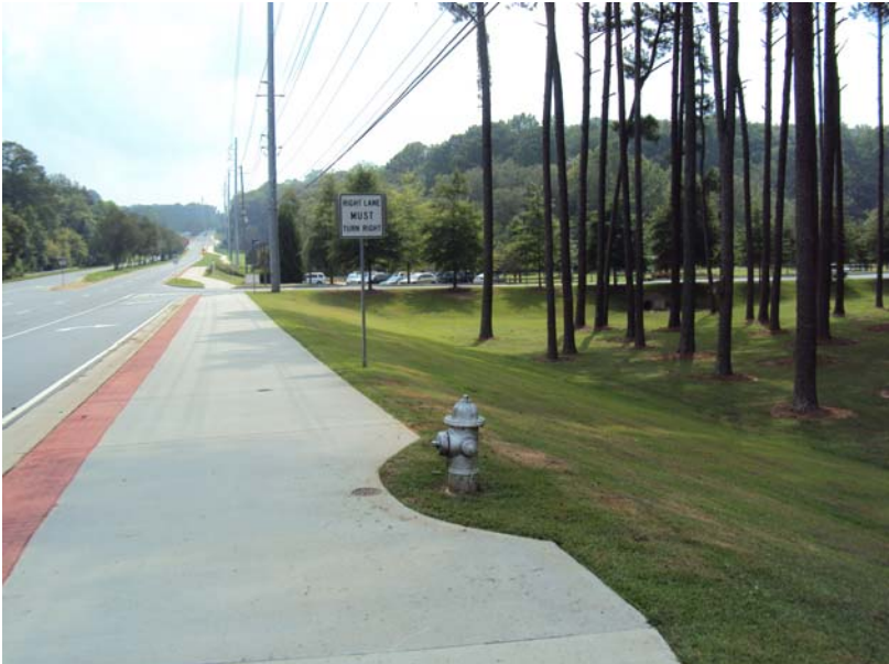
Figure 7: 5 Foot Sidewalk with Stained Concrete Strip
